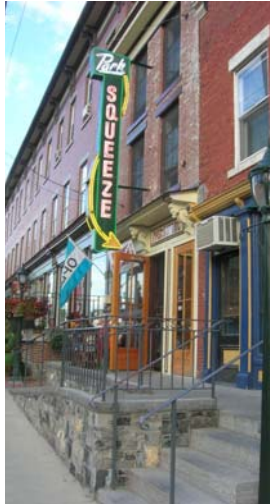
Example of limited and appropriate use of neon in an historic village
