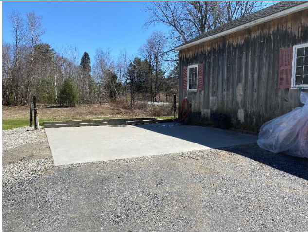
Photo 13: Equipment Wash Area
