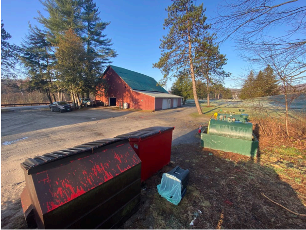
Photo 1: Stowe Country Club Maintenance Facility facing southwest toward equipment storage barn
