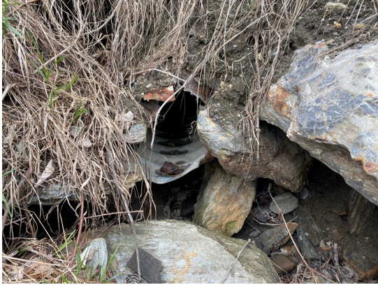
Photo 13: 12 inch Corrugated Metal Culvert leading to the West Branch Little River
