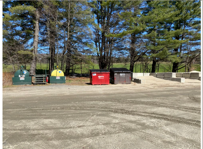
Photo 8: Two 350-gallon gasoline and diesel fuel ASTs
