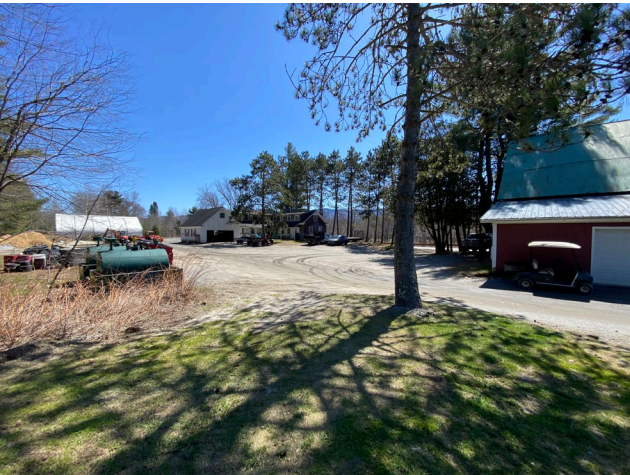
Photo 3: Stowe Country Club Maintenance Facility facing southeast toward Olsen House
