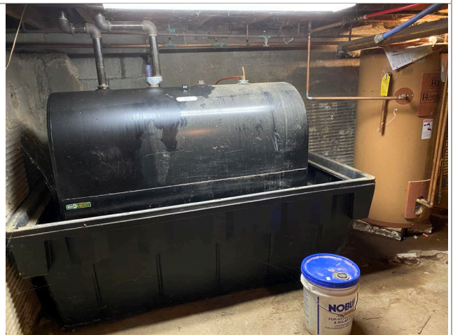
Photo 10: 275-gallon heating oil AST within secondary containment in Olsen House basement
