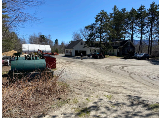
Photo 2: Two 350-gallon gasoline and diesel fuel ASTs
