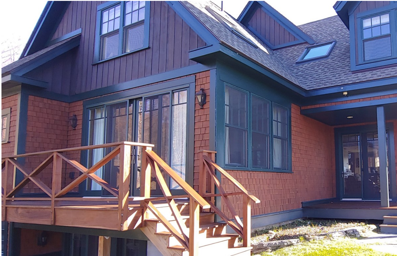
PROPOSED WINDOWS AND DOORS TO MATCH EXISTING MARVIN GREEN CLAD EXTERIOR WINDOWS AND DOORS
