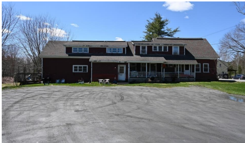
Figure 18. View of the historic house near with the River’s Edge Subdivision Development Project, in Stowe, Lamoille County, Vermont, looking westwards.
