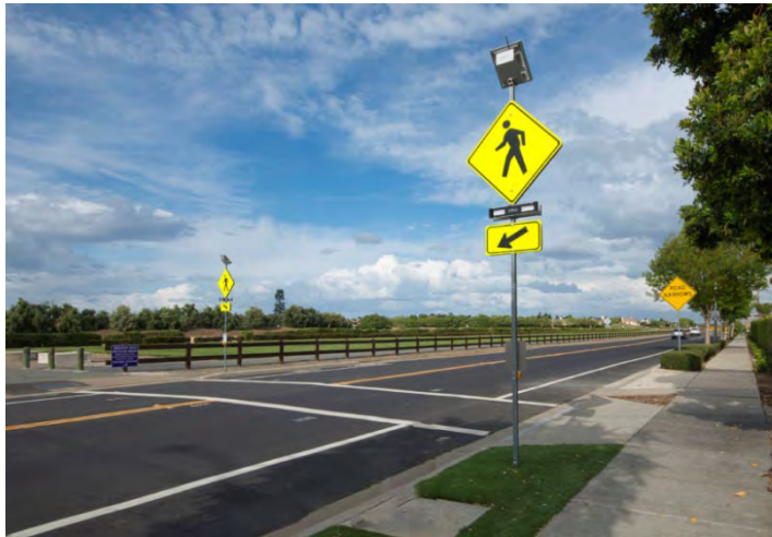
Rectangular Rapid Flashing Beacons (RRFB) (Image Source: Aailed Technologies Corp)
