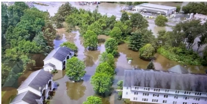
Figure 1-3 Mann’s Meadow apts. in Jeffersonville after July 2023 flooding
