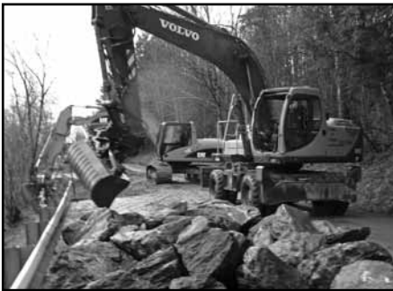
River Road Embankment Repair by Stowe Highway
