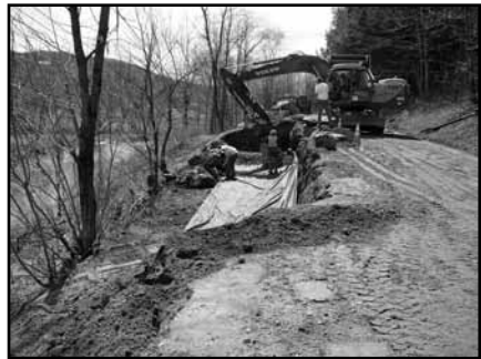
River Road Embankment Repair by Stowe Highway
