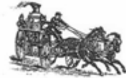
STOWE FIRE DEPARTMENT
