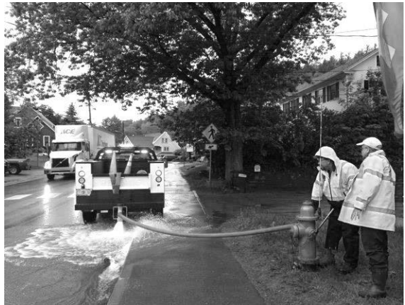
Water Department employees Al Ross and Richard Griffin flushing hydrants.
