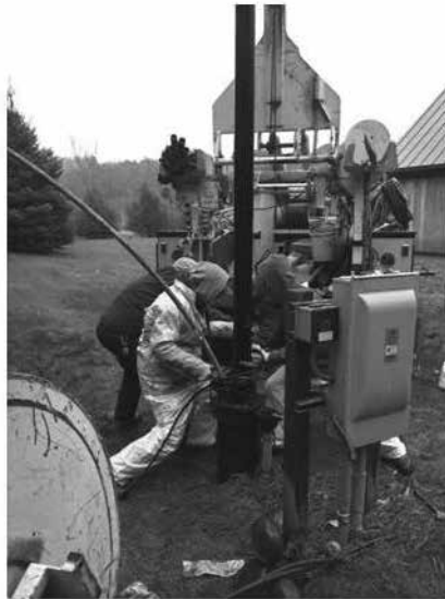
Village Green Well Pump Replacement
